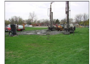
Drilling for new geothermal wells at Madison.
